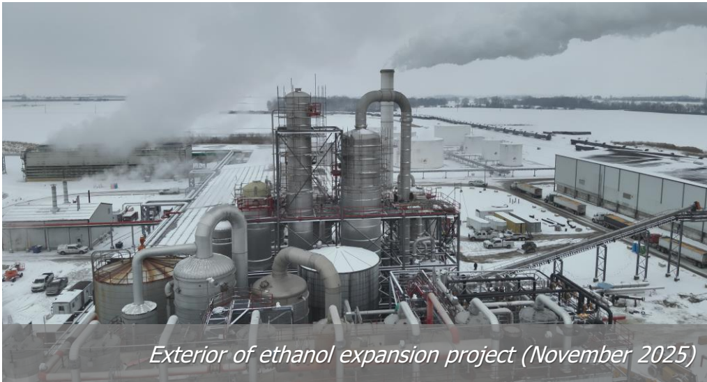
Exterior of ethanol expansion project (November 2025)
